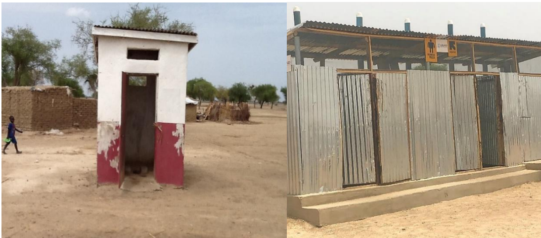
Figure 1 and 2: examples of latrines/toilet blocks in a displacement camp, not necessarily those built and maintained by the IRC.
