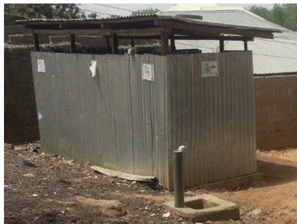
Figure 25: Cross flow ventilation does not circulate air through the pit but provides more air circulation for higher temperatures, Photo: Julien Graveleau
