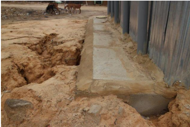
Figure 9: Soil erosion and collapse after rain events due to improper backfilling of excavated pits
