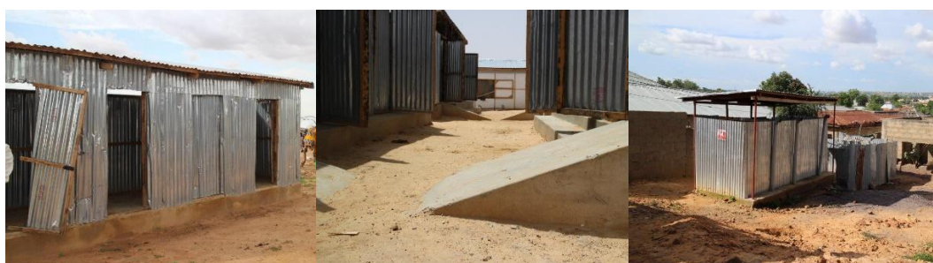
Figure 33: Latrines inaccessible by disabled and elderly include high steps (left), steeply sloped ramps (middle), and uncleared or steep areas (right)
