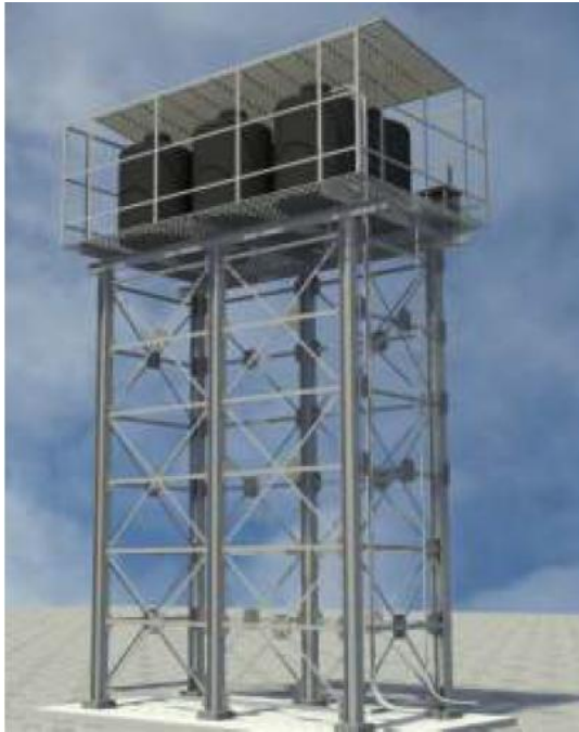
Figure 53: 24,000 L PVC tanks on 12 m stanchion
