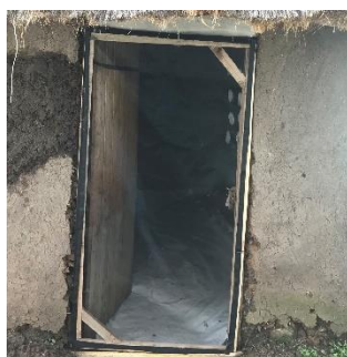
Figure13: Self-closing wood framed Velcro screened door
