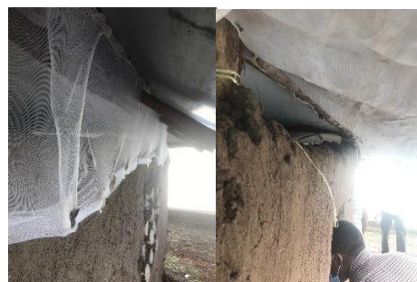
Figure 14 & 15: Unscreened eaves vs Screened Eaves
