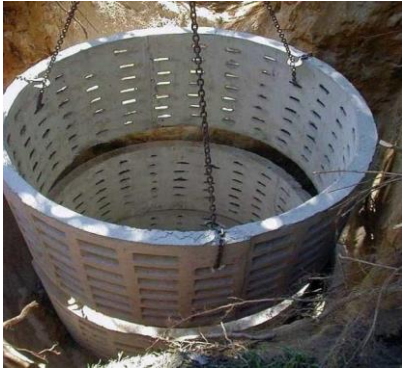
Method of installation of the treatment plant
