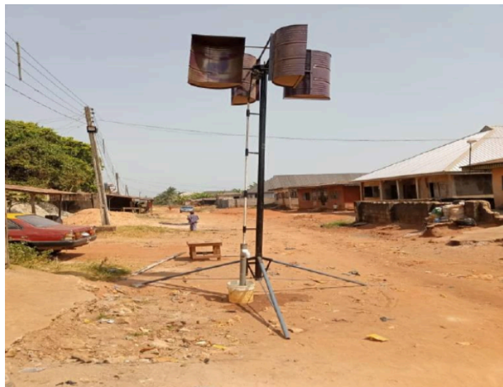
Figure 5.1. A typical very low cost, DIY, Savonius VAWT [1]
