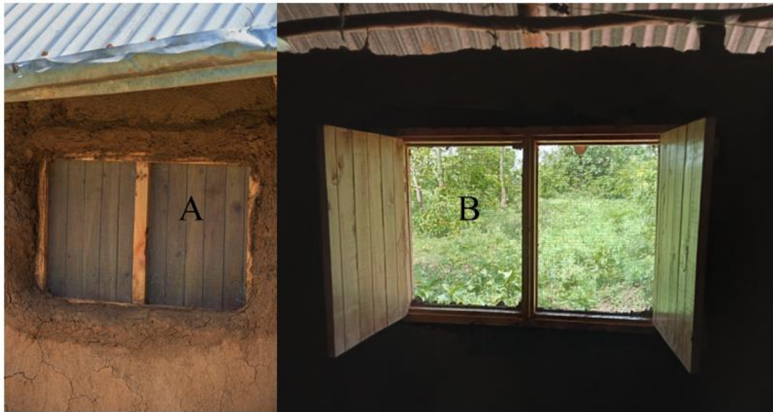
Figure 2: Image of screened windows, A is a closed window with image taken from outside of the house while B is an open window, image taken inside the house.
