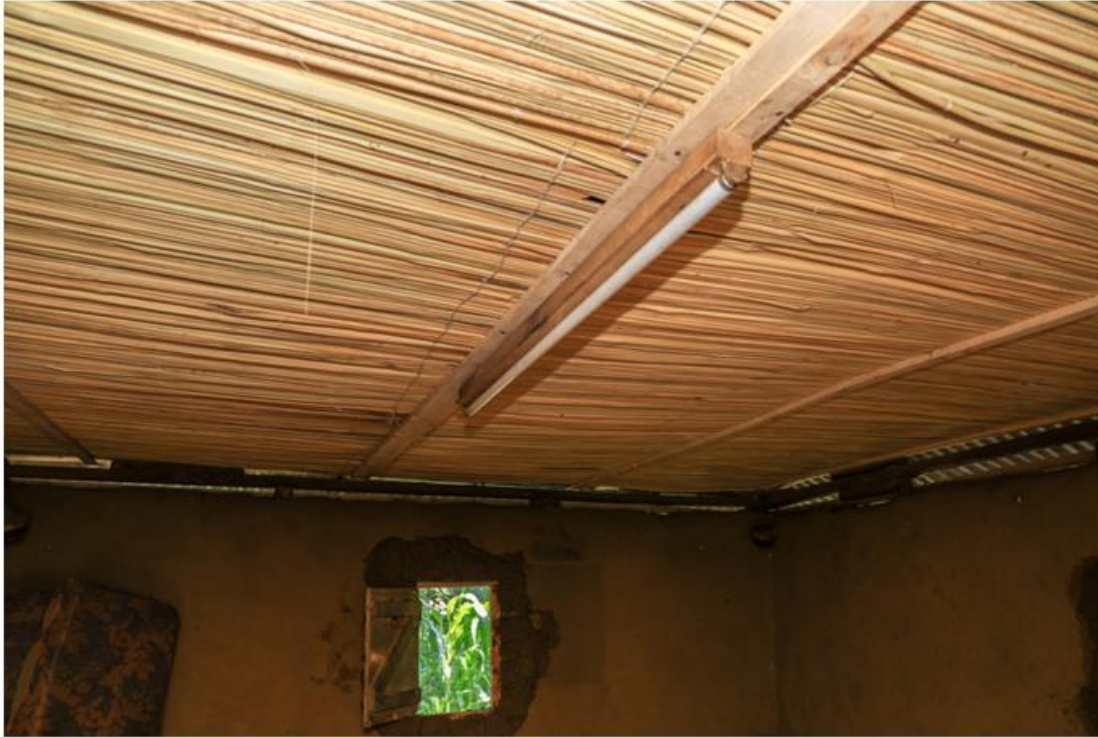
Figure 4: Image of mat ceiling
