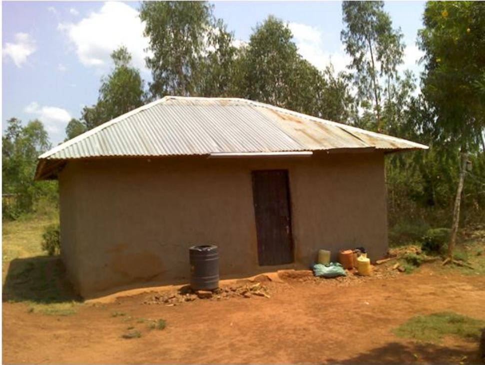
Figure 1: Picture of a typical house with iron roof and smeared mud wall in rural western Kenya.
