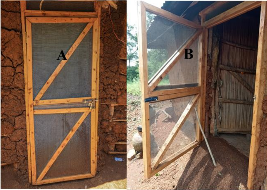
Figure 5: Image of screened doors, picture A showing closed screened door while B shows and open screen door.
