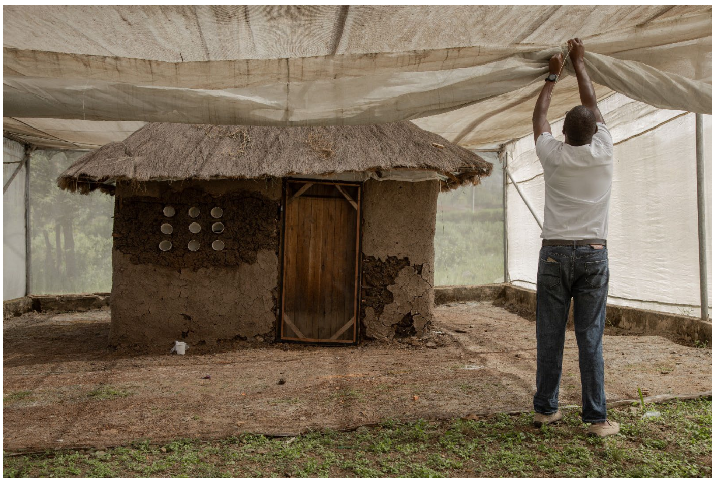
Figure 7: Modified hut with screen door and screened eaves
