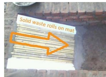
Fig. 4 shows bamboo sieve used to ensure collection of solid waste in chamber 2
