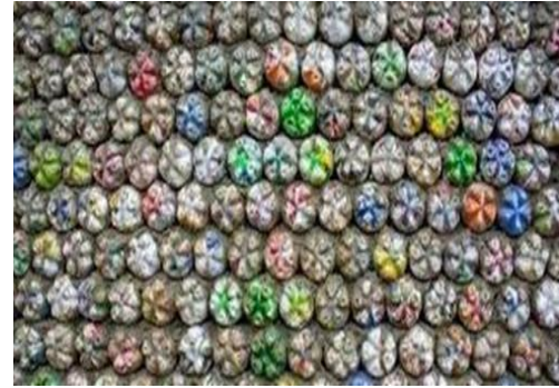
Fig. 3 Plastic bottles which have been set in concrete to form a bottle structure
