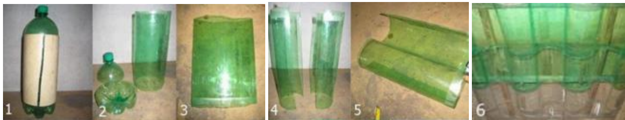
Fig. 6 illustrates the method of utilization of empty plastic bottles for construction of roof
