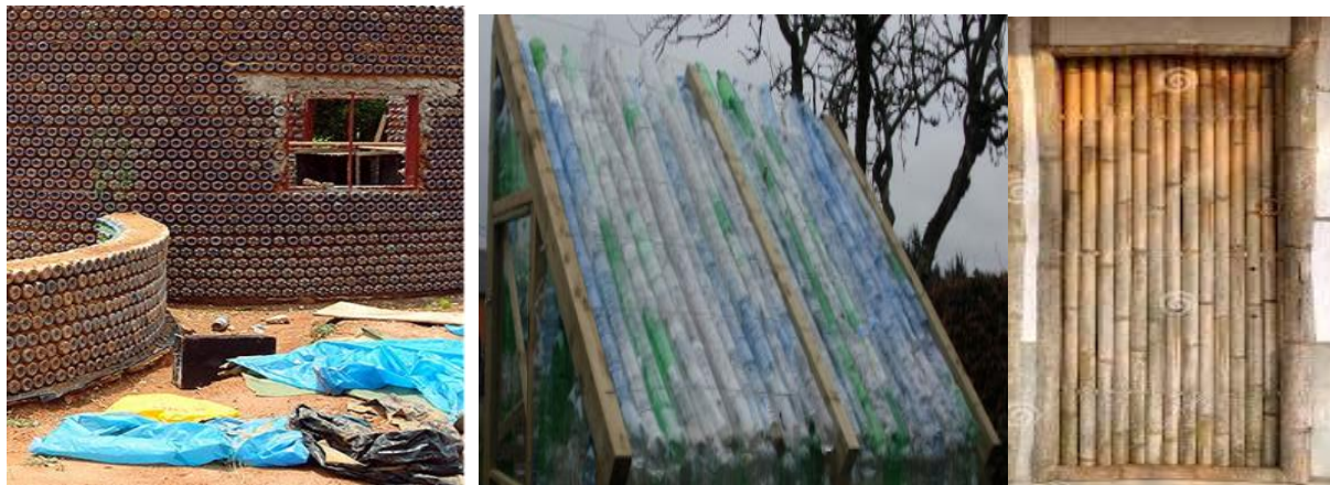
Fig. 7 Diagram illustrating the different parts of a super structure A. Wall structure constructed using used filled plastic bottles, stacked on their sides and bound together with mud or a cement mix, creating solid walls; B. Roof structure with Bamboo and Plastic Bottles; C. Shutters for door is made of bamboo
